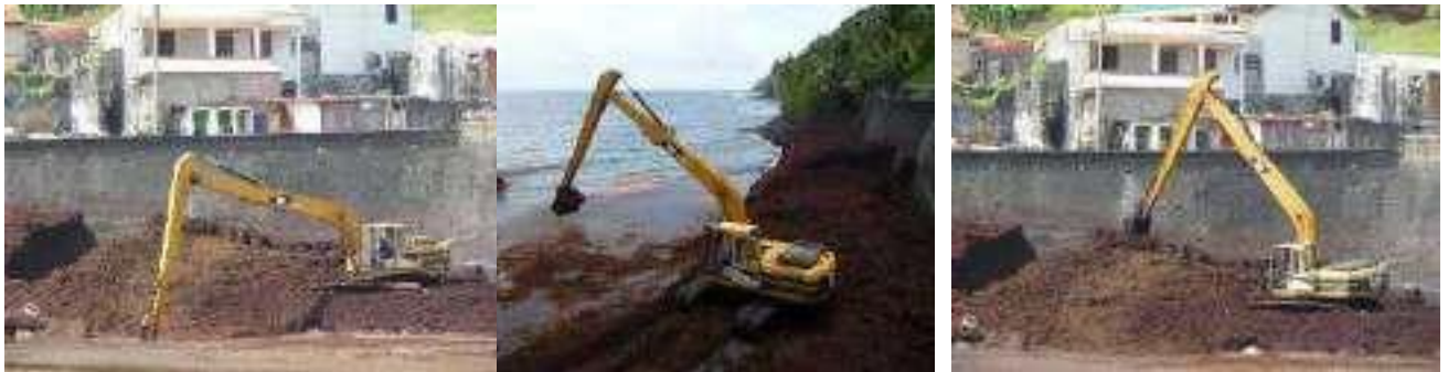
Figure 6: Harvesting sequence using a long-reach excavator
