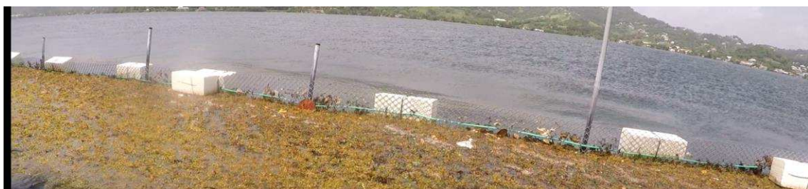
Figure 28: Polystyrene blocks installed in the Baie du Robert.
