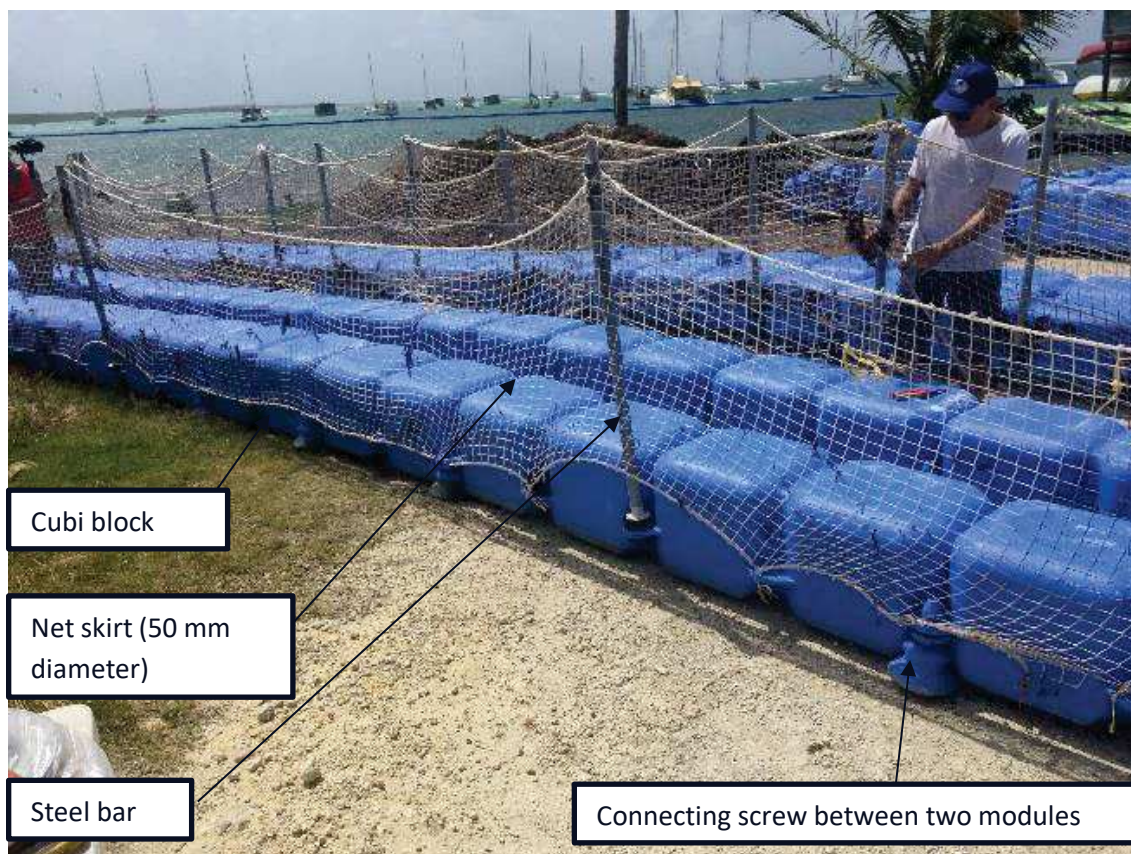
Figure 23: View of a barrier being assembled
