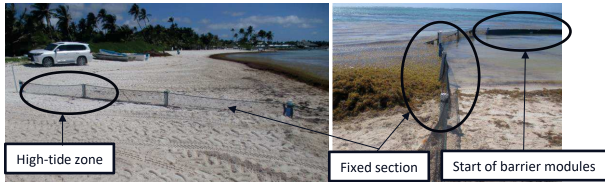
Figure 12: Illustration of a barrier set-up from the beach – AlgeaNova barrier.
